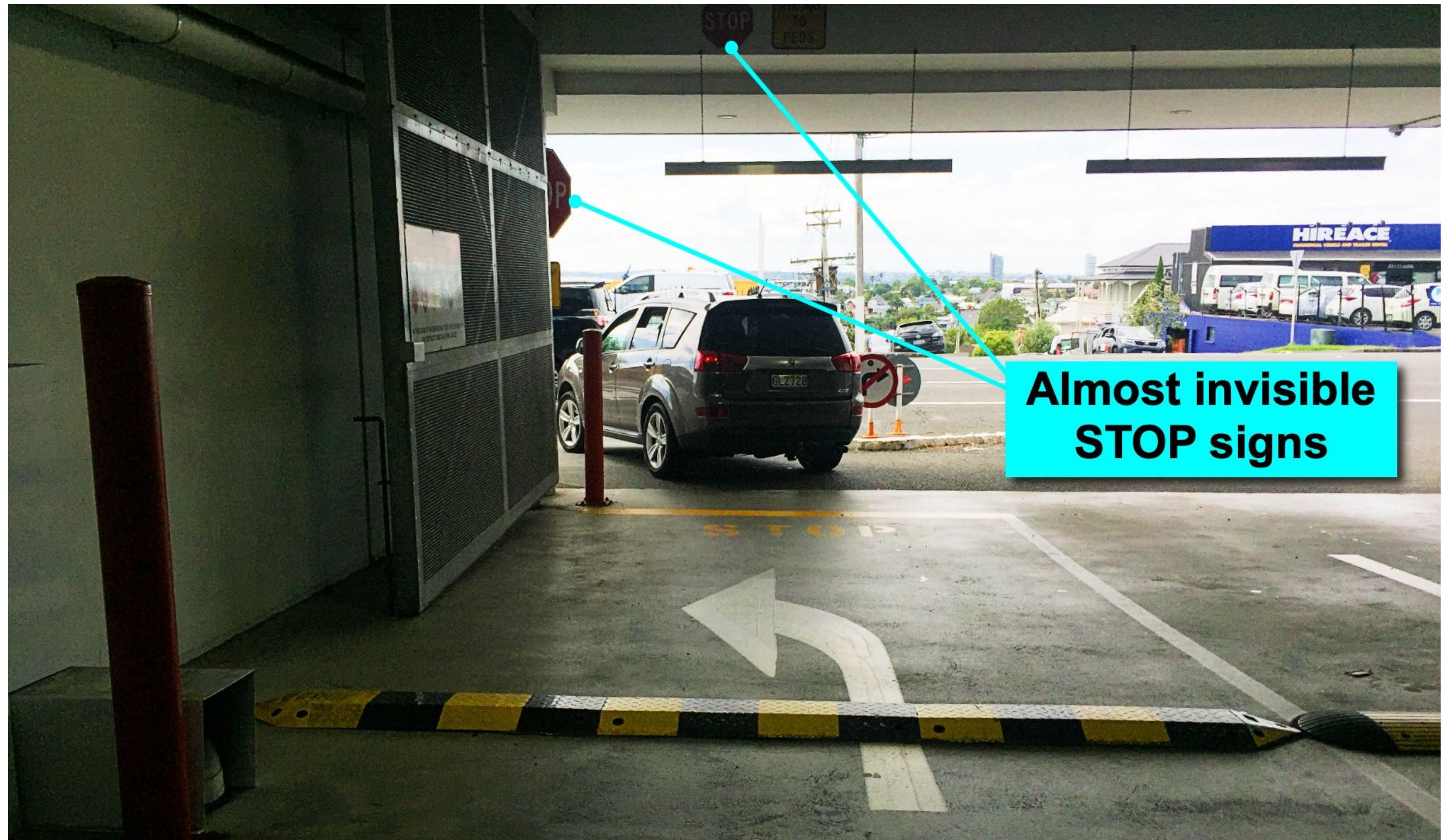
Almost invisible STOP signs and poorly placed judder bar does nothing to control traffic and puts pedestrians in danger.
